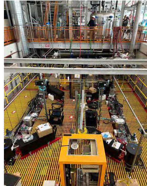
Cryostat welded closed and cabling installed
